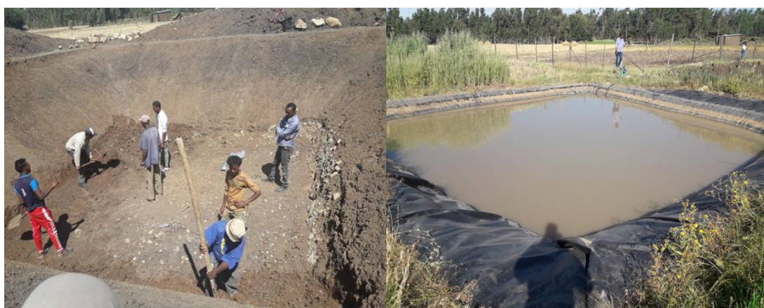
Fig 2:- Water harvester pond constructed
