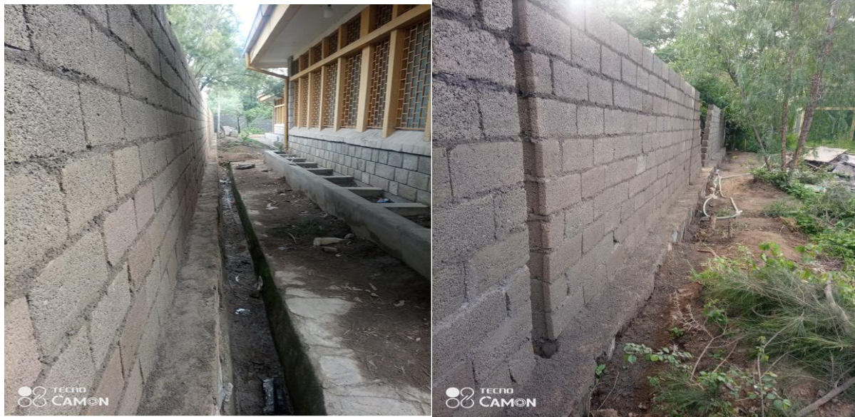
Figure 1. hundred meter fences constructed at Batu center on station
