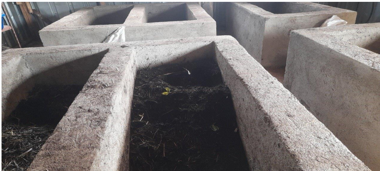
Figure 14: Construction of vermiculture center
